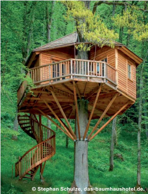
Figure 2.1 Unique construction: at the Baumhaushotel Seemühle, the 250-year-old oaks are holding some of the treehouse in 14 m height.
