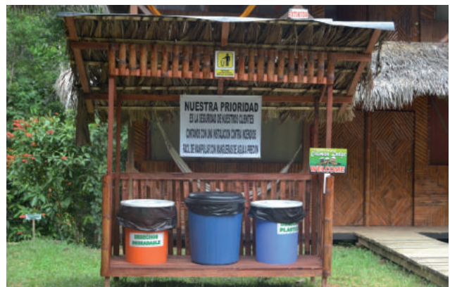
Figure 2.24 After receiving technical assistance from the Rainforest Alliance, the managers of this lodge in the Cuyabeno Wildlife Reserve built receptacles for the separation and recycling of solid waste.
